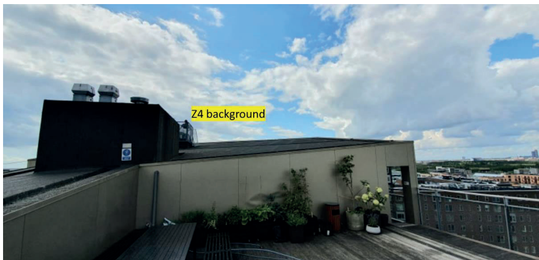
Figure 16. Z4 sensor installed at the background site on top of one residential building at Prismehaven area.
